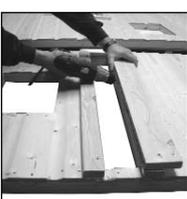
4 Fit handle. Place in the centre of the board. Fix using 4x 12mm black screws. Repeat for other shutter.
