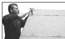
6 To obtain a neat finish at the corners, the felt will need to be carefully cut to enable one piece to be folded and sit under the other taking care not to cut too far - cut from the corner point of the felt to the outer edge of the felt. Trim any excess carefully.
