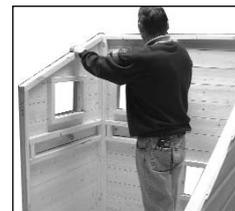
5 Place door panel 'G' into aperture. Drill and screw using 2x 60mm screws each side. (To secure the side with the door hinge, drill through the small rectangular panel).
