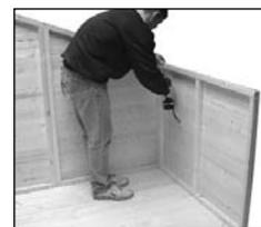
4 Place the other large window panel (F) next to the one already placed (B). Drill and screw using 2x 60mm screws.
