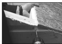
4 Lay another piece of roof panel (Q) into position ensuring it is flush with the previous panel. Fix using 3x 40mm nails at each short side and 3x 40mm nails in EACH roof panel along the roof bearer. Repeat.
