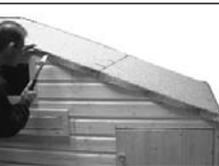
4 Nail along the edge of the felt which overlaps the previous felt into the roof panel. Secure using felt nails at approx. 100mm intervals.
