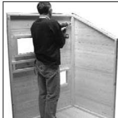
2 Place small plain angled panel 'D' next to the large plain panel 'C'. Drill and screw using 2x 60mm screws.
