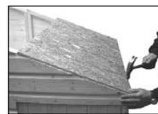
2 A roof bearer (P) needs to be placed beneath the joints of each roof section (Q). The roof bearer should be flush with the top of the framework of the side panels. Near the top of the side panels where the roof panel finishes, drill a hole. Repeat for other side.
