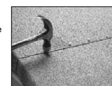
5 Place the small roll of felt onto the remaining part of the roof. Secure as previous.
