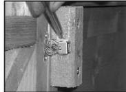
3 Close the door and attach the door catch together and mark the required position of the door catch housing. Secure using 2x 25mm screws.
