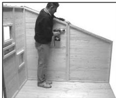
3 Place small rectangle panel 'E' along the shortest side of the floor (opposite the large window panel). Drill and screw using 2x 60mm screws.
