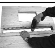
3 Fit observation port shutter into aperture. Place the board H (with hinge already fitted) into the aperture of the relevant size panel, ensuring the hinge is at the bottom. Secure into place using 14x 20mm screws for the long gun port board and 10x 20mm screws for the short.
