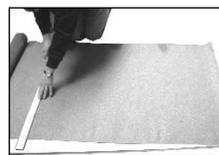
2 Lay one piece of felt along the bottom lowest edge. The felt should overhang each side by approx. 40mm. Secure the felt using felt nails at approx. 100mm intervals and nail directly down into the walls.
