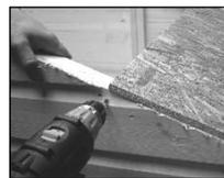
3 Fix a roof bearer (P) using the pre-drilled holes using 2x 80mm screws, one at either end.
