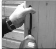
3. Place the front panel 'G' onto a flat level surface, outside facing up. Place the door into the aperture, ensuring that there is an equal gap between the edges of the door and the aperture. Screw into position using 6x 25mm screws.
