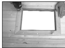
Drill and screw into place using 3x 25mm screws per long piece and 2x 25mm screws per short piece. Repeat for other 2 windows.
