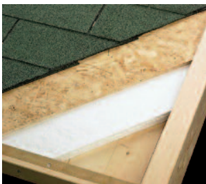
Roof insulation
